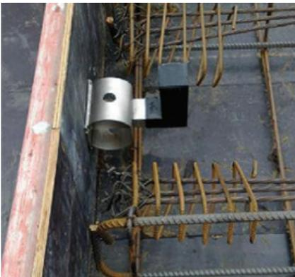
HLDQ-L30 Sleeve nailed to formwork
