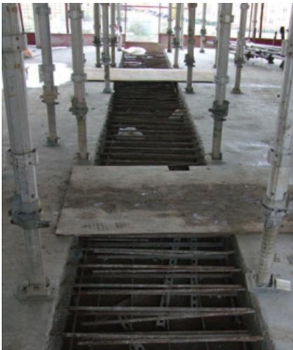
Pour Strips restrict site access, cause a trip hazard and delay progress on site
