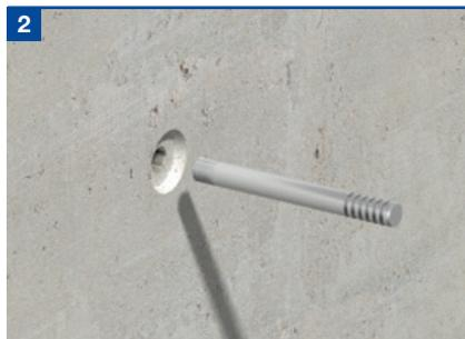
When concrete reaches sufficient strength, strike the formwork and remove nailing plate. Screw the dowel into the anchor.
