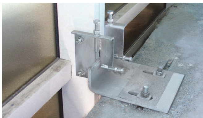
Fixing of a curtain wall system using HCW-B2 Brackets connected to HTA-CE Cast-in Channels
