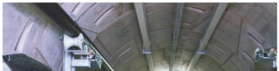
Curved Halfen Cast-in Channels in tunnel segments
