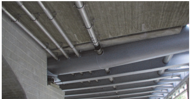
Fixings for drainage systems
