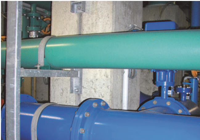
Pipe supports on vertical HZA Channels
