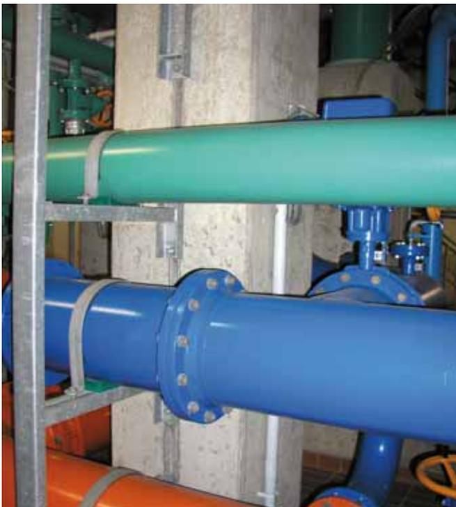
Pipe support using vertical cast-in channels
