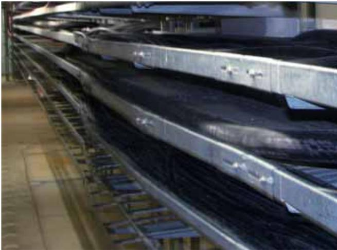
Stacked cable trays; by bolting to vertical serrated channels
