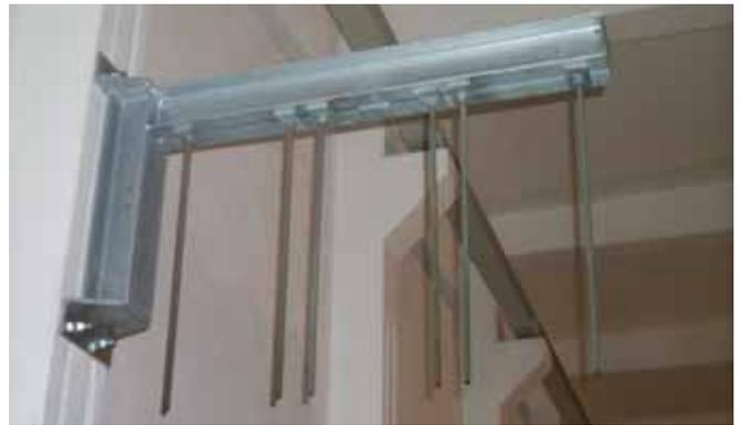
Cantilever for support of pipes mounted to vertical serrated channel
