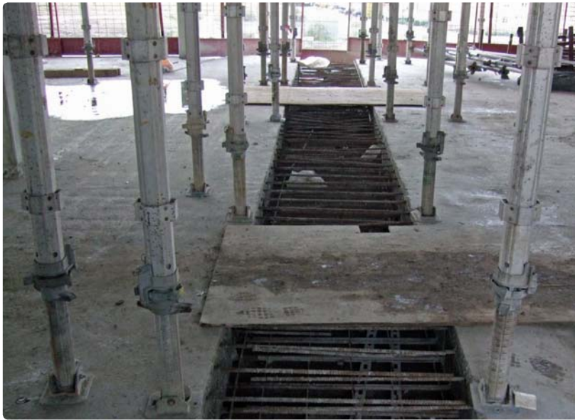
Above: Example of site access issues with an open pour strip.
