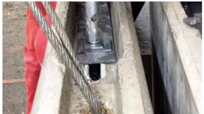
HVL-System with precast building components
