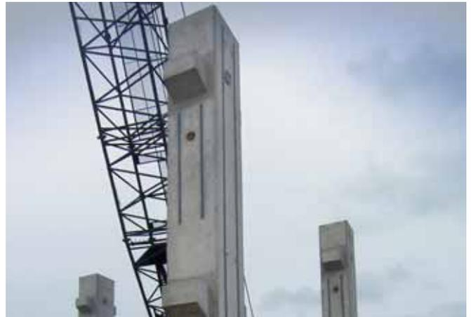
Vertical channels in columns to attach further components
