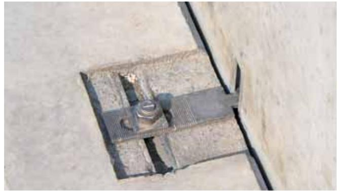
HALFEN HKZ Restraint tie with serrated washer
