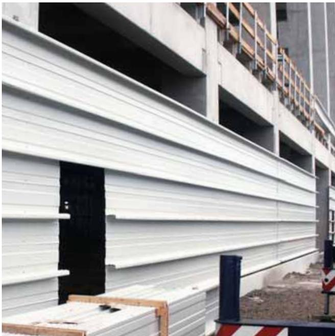
Façade fixed using HALFEN HTU Cast-in channels
