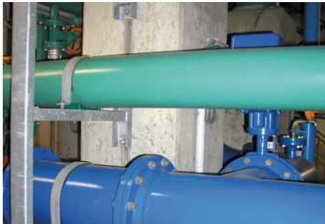
Pipe supports on vertical HZA-channels
