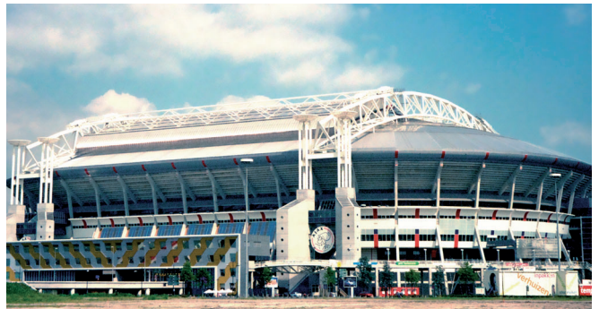
APPLICATION IN PRECAST ELEMENTS FOR STADIUMS
