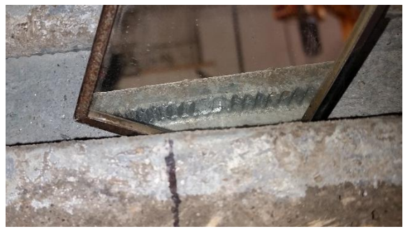
Figure 11 – Damaged Teeth inside the channel lip after longitudinal shear test
