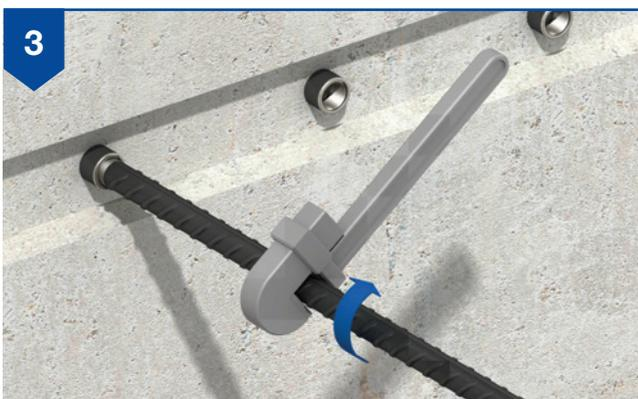
The RT parallel threaded reinforcing bar is rotated into the RT KSN Anchor and tightened using a wrench. No more than 2mm of thread should be left exposed on the bar. Fix the slab reinforcement and pour the concrete to complete the installation.
