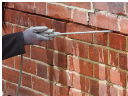
STEP 2 Clean out slots with a blow pump and apply HeliPrimer WB or flush with water.
