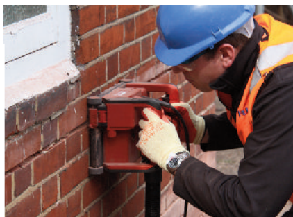
STEP 1 Cut slots into the masonry to a minimum of 500mm either side of the crack and to the specified depth.
