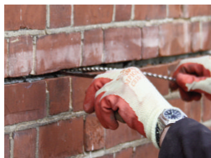
STEP 4 Using a finger trowel, or similar, push the HeliBar into the grout to obtain good coverage.
