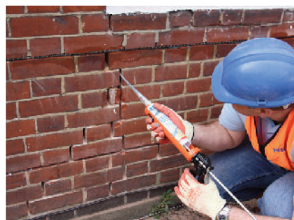
STEP 6 Repoint the mortar bed with a suitable mortar and make good the vertical crack with an epoxy-based weatherproof filler, e.g. CrackBond TE.
