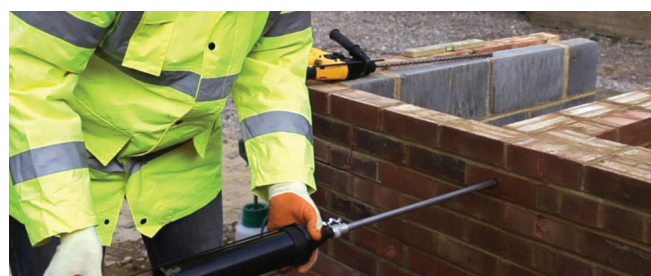
Inserting the grout-filled pinning nozzle, containing the CemTie, into the clearance hole
