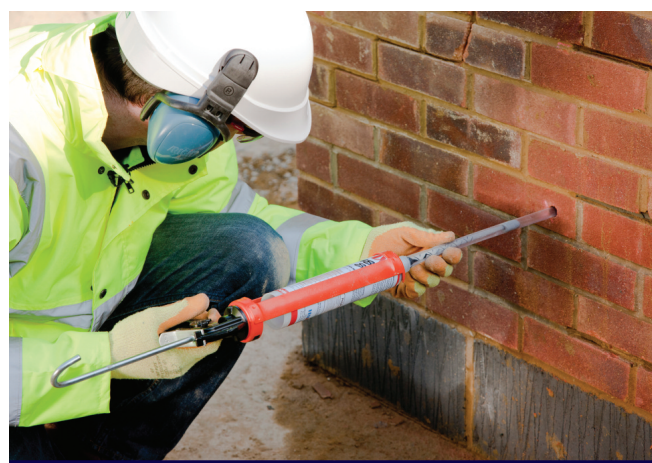
Injecting resin to complete the RetroTie installation
